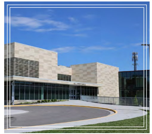
Bond 2016 funds helped renovate the Mill Creek Campus to accommodate growth of the Prairie Learning Center.
