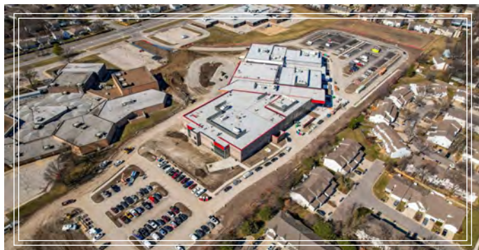
Santa Fe Trail Middle School, construction in progress
